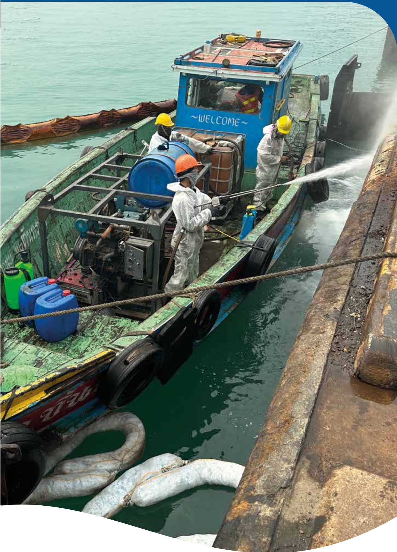
IMAGE: USING HIGH PRESSURE WASHING TO CLEAN PORT INFRASTRUCTURE, THAILAND
