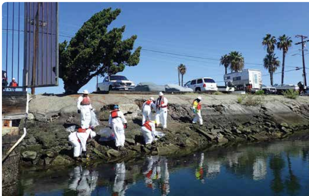
ISTRACE: Workers cleaning oil streaks from rip rap and pilings in marina
