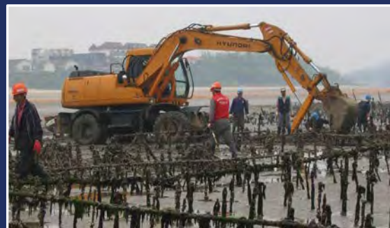
Removal of oiled mariculture facilities
