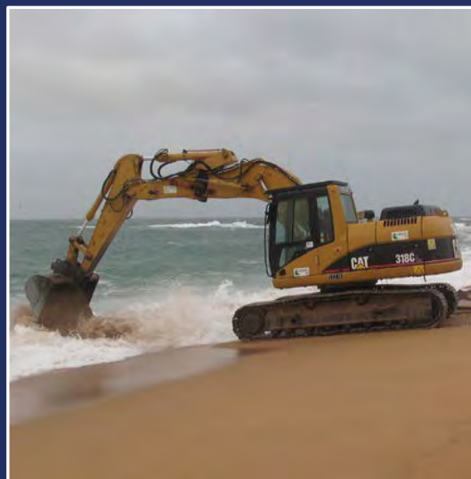
Moving lightly-oiled sand for cleaning by natural wave action (surf washing).
