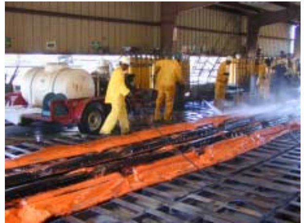
Decontamination of a section of the 9000+m of boom used
