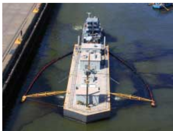
Skimming operations alongside the quay in Barbers Cut
