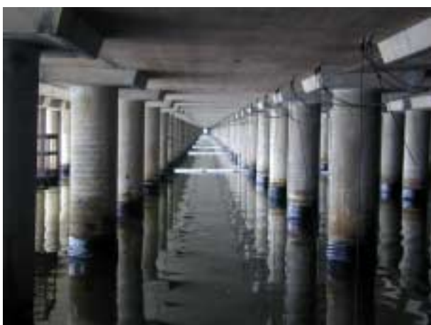
After the Flush. Barbers Cut Container Terminal quay is 1 mile long. Its supporting pillars were oiled
