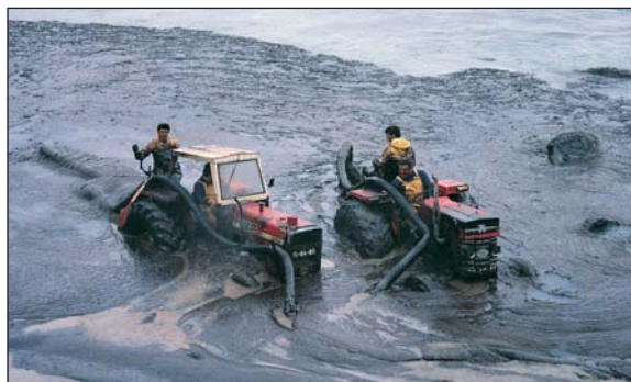
Left: removal of bulk oil from shorelines often calls for the use of locally-available non-specialized equipment. Right: the temporary storage and final disposal of recovered oil and debris is frequently a major component of any clean-up operation.
