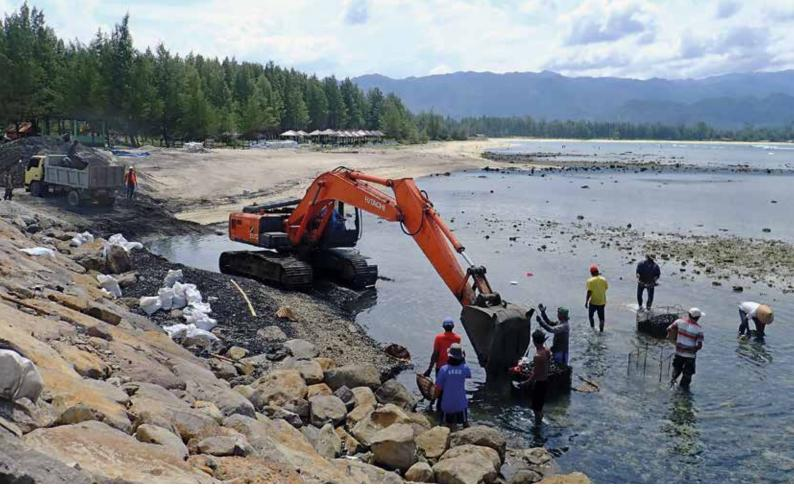
Mechanically assisted clean-up of coal in a lagoon, Indonesia
