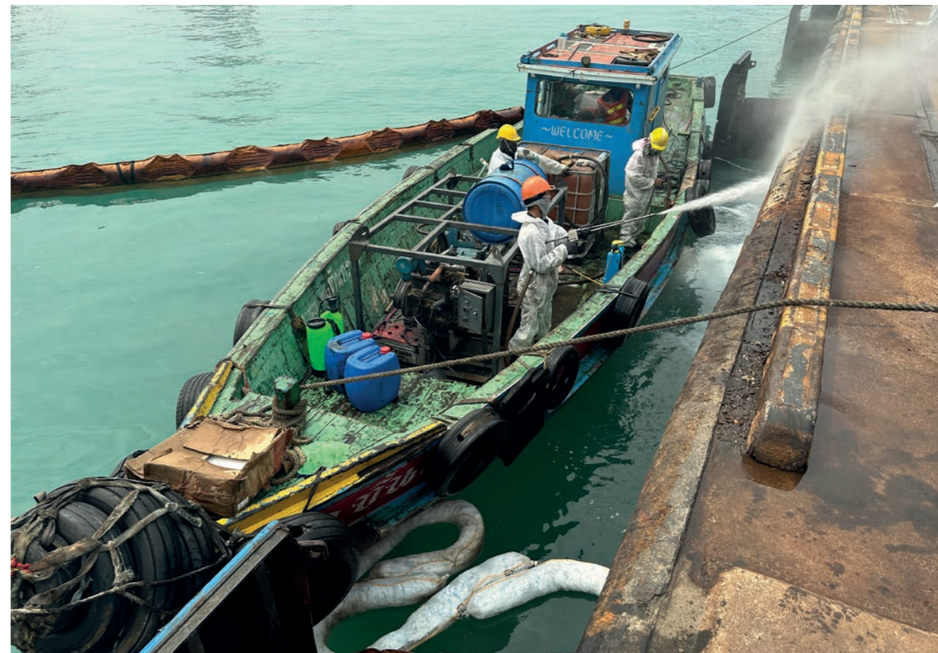
CONTRACTORS USING HIGH PRESSURE WASHING TO CLEAN SIDE OF PORT, THAILAND
