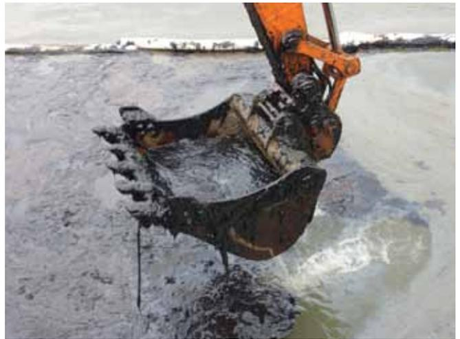
▲ Figure 21: Use of an excavator to recover highly viscous fuel oil. The concentration of recovered oil was maximised by instructing the operator to hold the bucket above the water surface for a short period, to allow entrained water to run off. This reduced the subsequent disposal costs at the expense of recovery efficiency.
